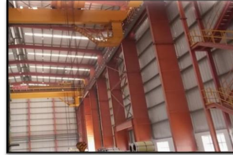
Use of Transparent Sheet for natural lighting in plant
